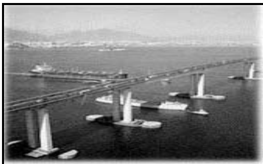
Fig.3 Aerial image of the Rio-Niteroi bridge in the Guanabara bay.
