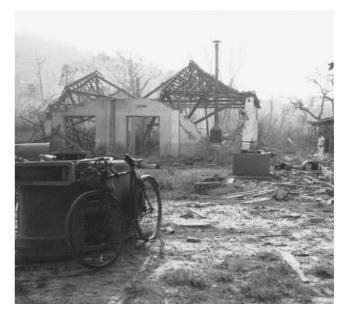
Fig. 2. Machine shop I. Picture taken 80 m from epicenter (obviously the bicycle belonged to the photographer).
