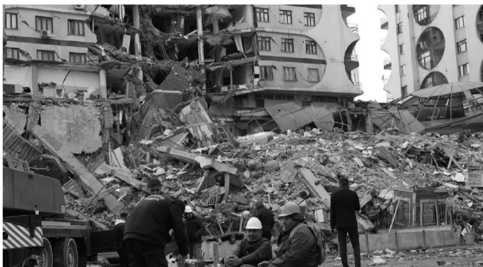
Figura 1. Earthquake damage in the city of Diyarbakir, Turkey in February 2023.
