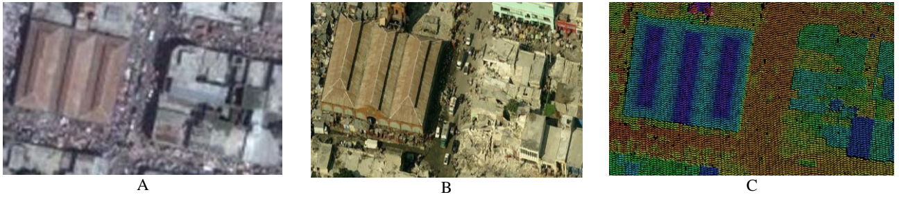
Figure 1. Comparison of aerial image and laser data of a damaged and an intact building. A. Pre-event aerial image; B. Post-event oblique aerial image; C. Post-event aerial laser data.
